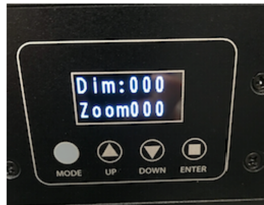
NO DMX CABLE CONNECTED
